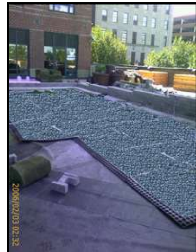
(L) Lightweight retaining walls and lighting wire. (M) 2' caliber trees (IMPORTANT! DO NOT EXCEED THE ROOF LOAD CAPABILITIES!) (R) Root barrier and green living roof panels are installed in preparation for the trees and growing media.
