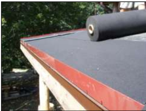
Left: Protection fabric being installed on top of a single ply TPO. GLTI Orange NY.
