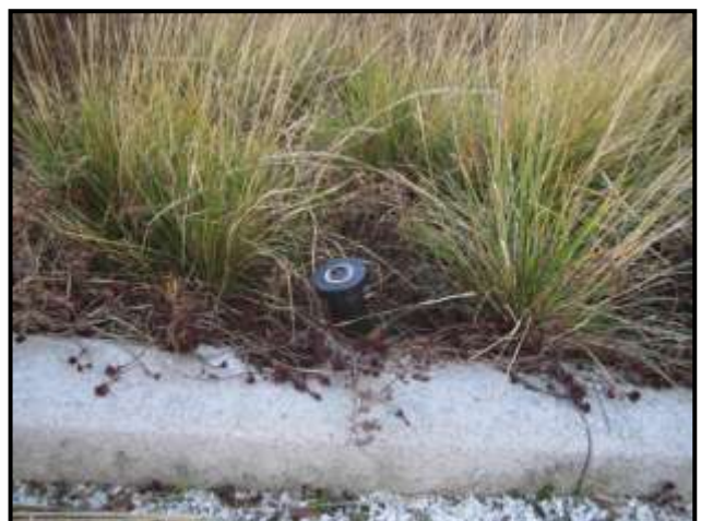
Above & below 6" pop ups were poorly chosen to irrigate an area that is blocked by a larger grass. The 6" pop up will NOT provide proper coverage overwatering and wasting water.
