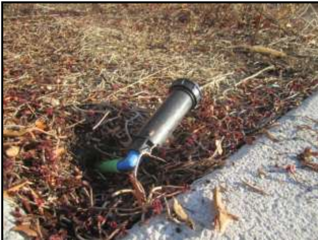
Above & below poor design showing a 6" pop up connected to flexible piping. If the head was placed on a riser it would be subject to breakage.
