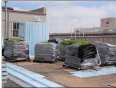
Left: Plywood is prepared to stage green roof pallets. Right: Pallets are staged on top of the plywood to protect the insulation and waterproofing
