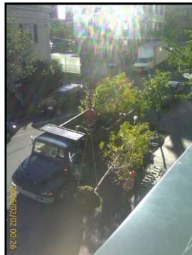
(L) Lightweight retaining walls and lighting wire. (M) 2' caliber trees (IMPORTANT! DO NOT EXCEED THE ROOF LOAD CAPABILITIES!) (R) Root barrier and green living roof panels are installed in preparation for the trees and growing media.
