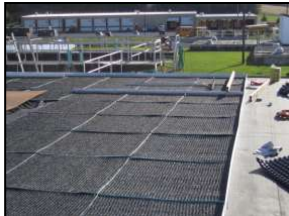
Install protection fabric / slip sheet as per specification *not required with CTEM
