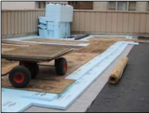
Left: Plywood is prepared to stage green roof pallets. Right: Pallets are staged on top of the plywood to protect the insulation and waterproofing
