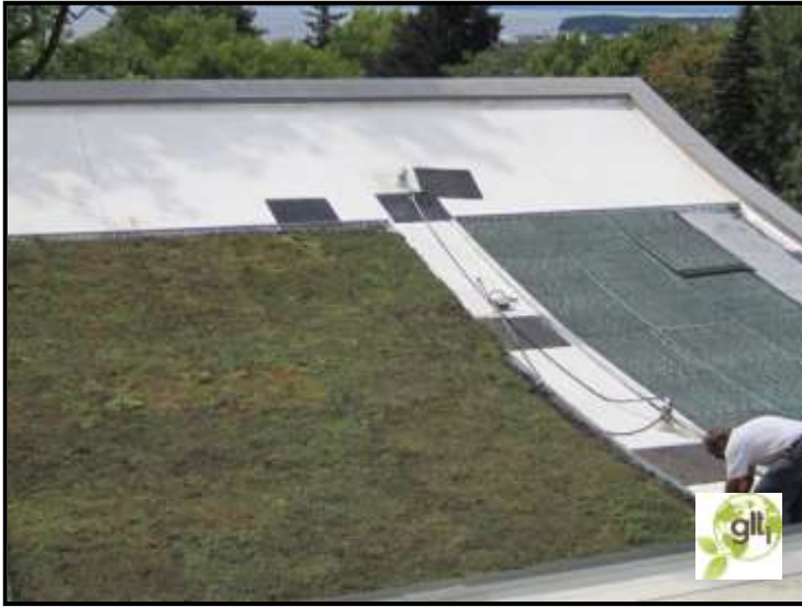
The GLTi system displays flexibility, easy to cut curves, angles and account for undulations. No media falls between the seams Left: GLTi Right: Live Roof
