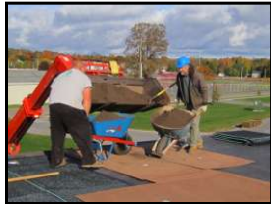
Protection Boards to Maneuver Engineered Growing Media
