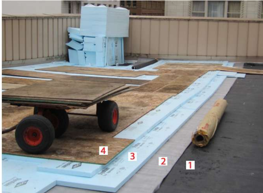
Portland Oregon, Protected Assembly in Preparation to Accept the Pre-Grown Patented GLTI Green Living Roof Panels
