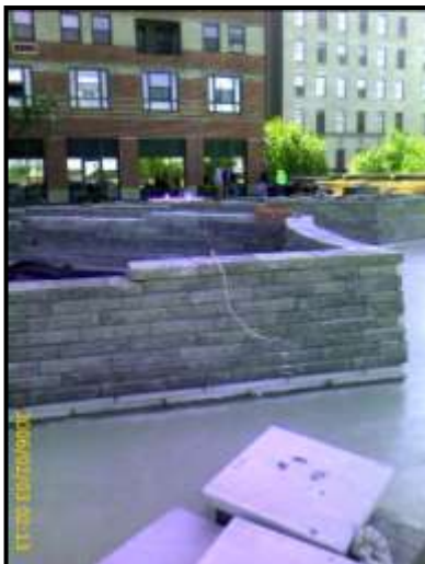
(L) Lightweight retaining walls and lighting wire. (M) 2' caliber trees (IMPORTANT! DO NOT EXCEED THE ROOF LOAD CAPABILITIES!) (R) Root barrier and green living roof panels are installed in preparation for the trees and growing media.
