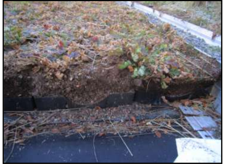
Media Quality & Termination Details Left: GLTi Right: Live Roof
