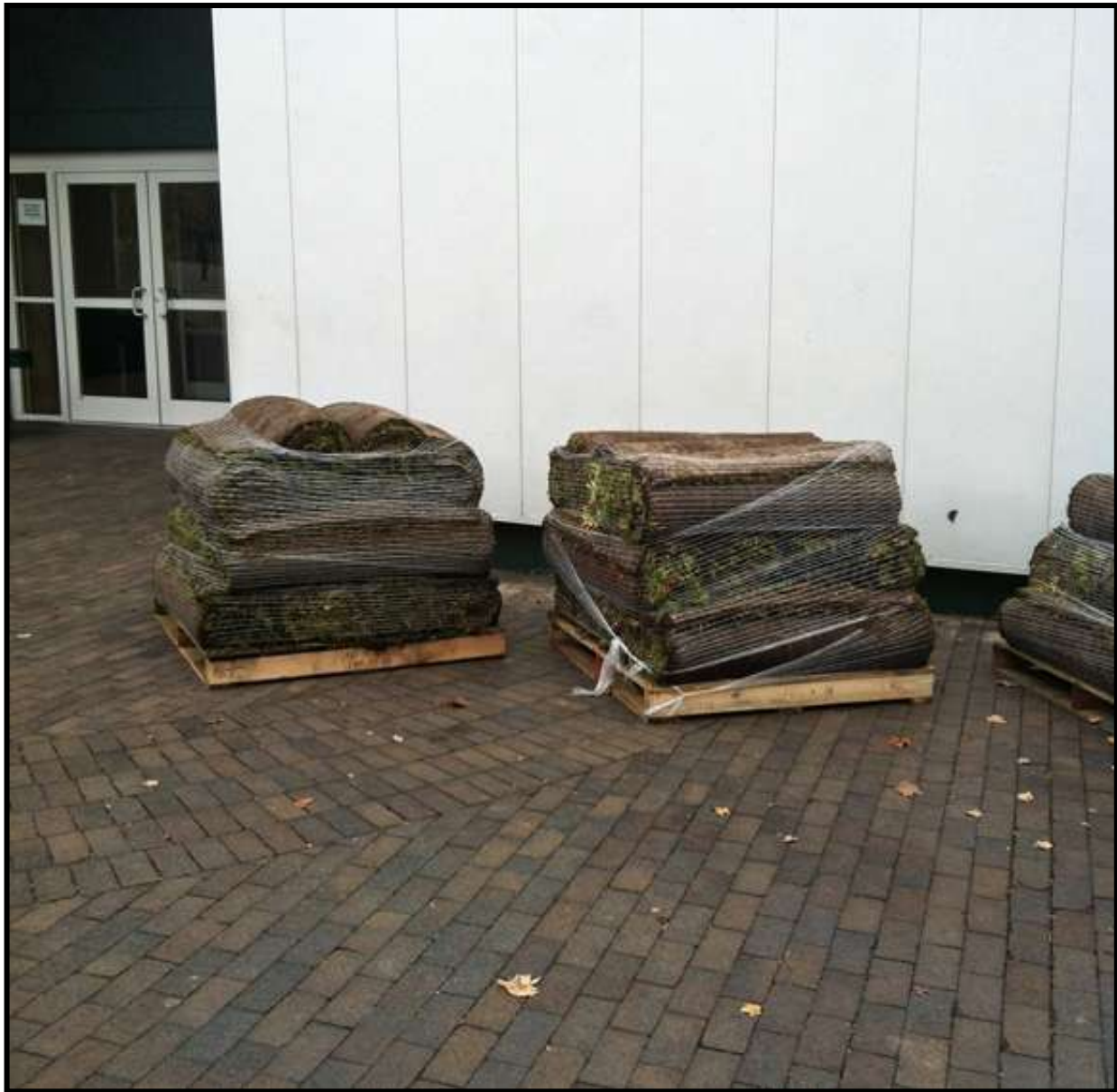
Mature sedum rolls preparing to be lifted to the roof. Notice the air flow mesh that keeps the rolls securely on the pallet. The vegetative material should never be delivered in plastic wrap. In some cases if extra security is needed temporarily wrap the pallet in plastic until it is secured on the roof.
