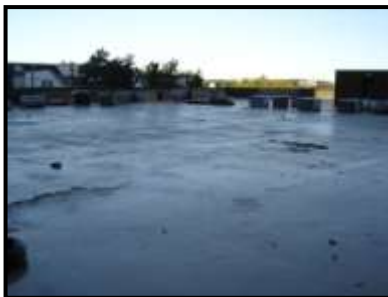
(L) Prep the area and mark out the planting beds. (M) Stage pallets of materials (IMPORTANT! DO NOT EXCEED THE ROOF LOAD CAPABILITIES!) (R) Root barrier, wall construction, irrigation and lighting preparation.
