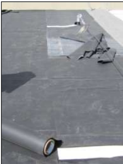
(Fig. 1 Root Barrier Overlap)
