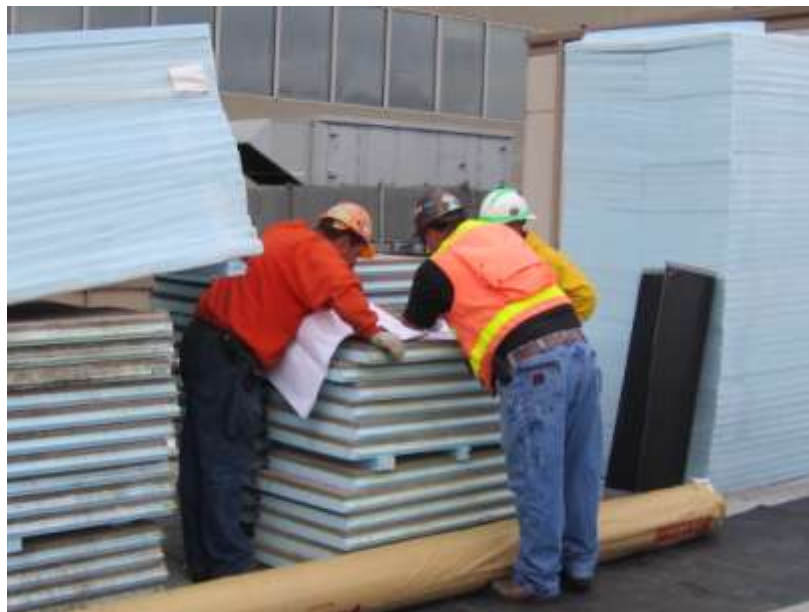
Communicate with co-workers to prevent injury and improve the flow of work. Above project managers and co-workers review the plan to move vegetation.
