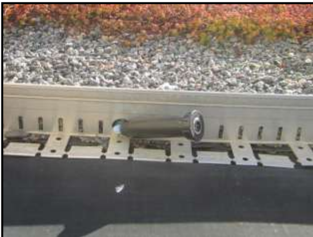
Above & below poor design showing a 6" pop up connected to flexible piping. If the head was placed on a riser it would be subject to breakage.
