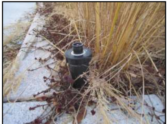
Above & below 6" pop ups were poorly chosen to irrigate an area that is blocked by a larger grass. The 6" pop up will NOT provide proper coverage overwatering and wasting water.
