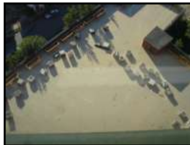
(L) Prep the area and mark out the planting beds. (M) Stage pallets of materials (IMPORTANT! DO NOT EXCEED THE ROOF LOAD CAPABILITIES!) (R) Root barrier, wall construction, irrigation and lighting preparation.
