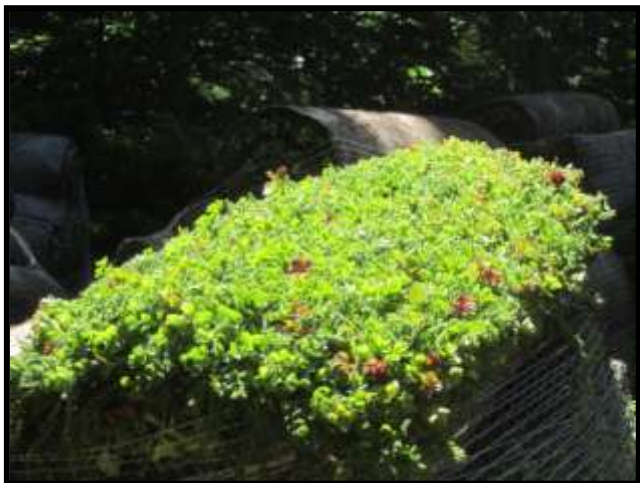
Sedum rolls stored in the shade in preparation for installation.
