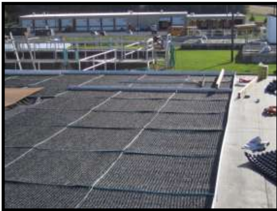
Protection Fabric, Edging and the Green Living Roof Panels in Place
