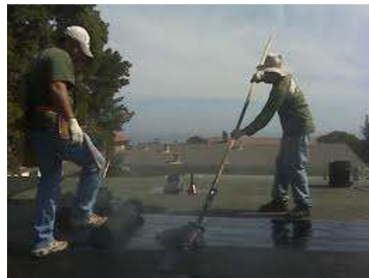
Hot Mop being applied to layers of felt and reinforced fiberglass
