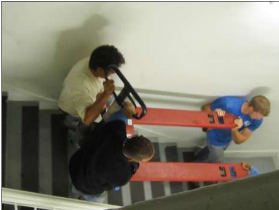
A Pallet Jack had to be removed from the roof 8 stories high via a staircase because it was forgotten after the crane was disassembled.
