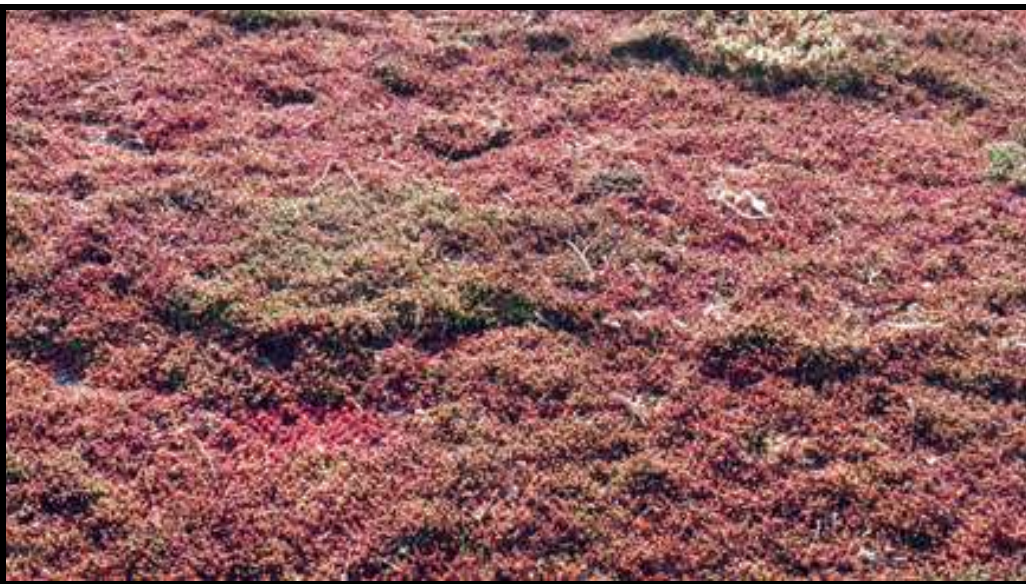
Below - Green Living roof (close up) with bioSoil (winter) showing no voids or erosion
