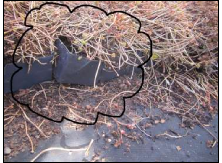
The GLTi system displays flexibility, easy to cut curves, angles and account for undulations. No media falls between the seams Left: GLTi Right: Live Roof
