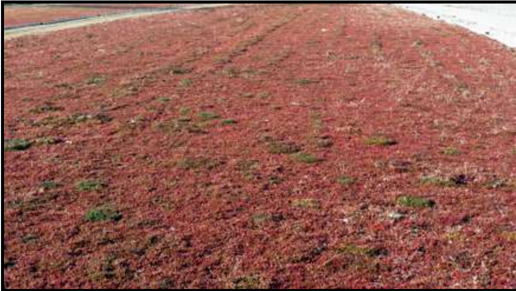
Below - Green Living roof (close up) with bioSoil (winter) showing no voids or erosion
