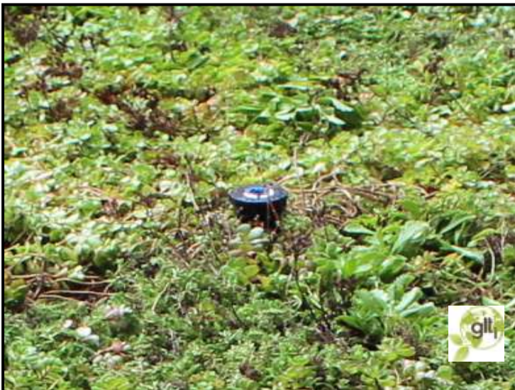
Because of the GLTi flexibility, irrigation can be installed directly under the green living roof panels with NO need to modify the system to stabilize irrigation heads.
