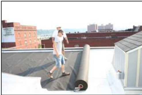
Left: Protection fabric being installed on top of a single ply TPO. GLTI Pittsburgh PA.
