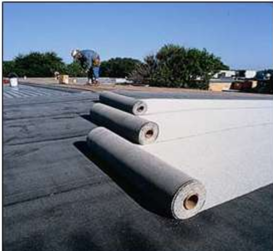
Fig 1 Picture by National Roofing partners
