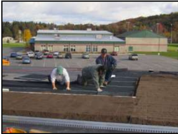
Growing media installation
