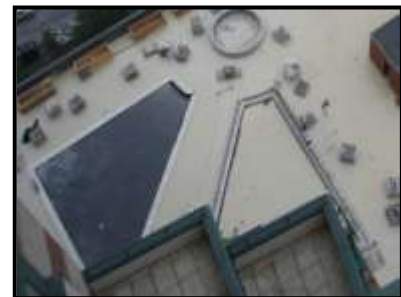
(L) Prep the area and mark out the planting beds. (M) Stage pallets of materials (IMPORTANT! DO NOT EXCEED THE ROOF LOAD CAPABILITIES!) (R) Root barrier, wall construction, irrigation and lighting preparation.
