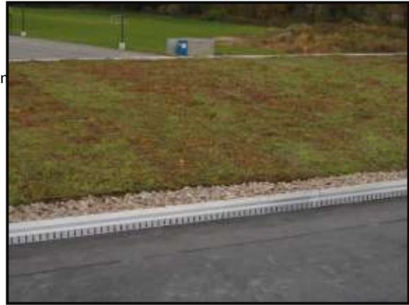
Sedum blanket installation
