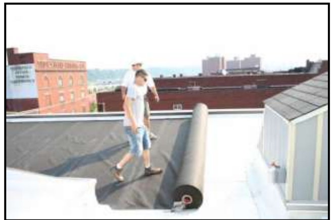
Install protection fabric / slip sheet as per specification *not required with CTEM
