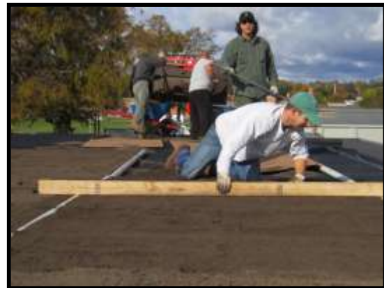
Engineered Growing Media, Screed to Depth
