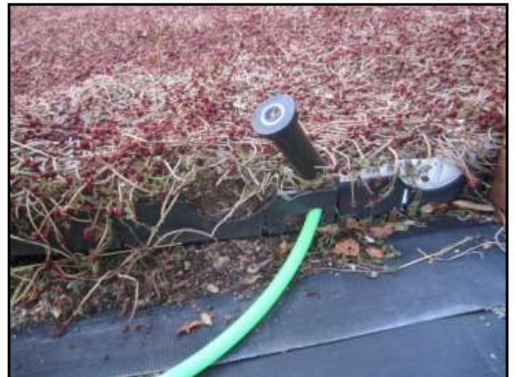
The tray displays an inability to properly irrigate vegetation without modifying the tray, and this compromises its integrity and function.
