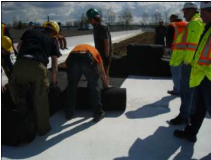
Left: Inspections to the waterproofing prior to the protection fabric being installed on top of a single ply TPO. GLTI Sysco Foods, Vancouver BC, 68,000 ft 2
